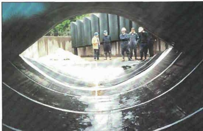
6 Membrane installed in hydro duct
